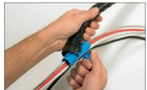
Place the applicator tool in one end of the Helawrap cable cover.
